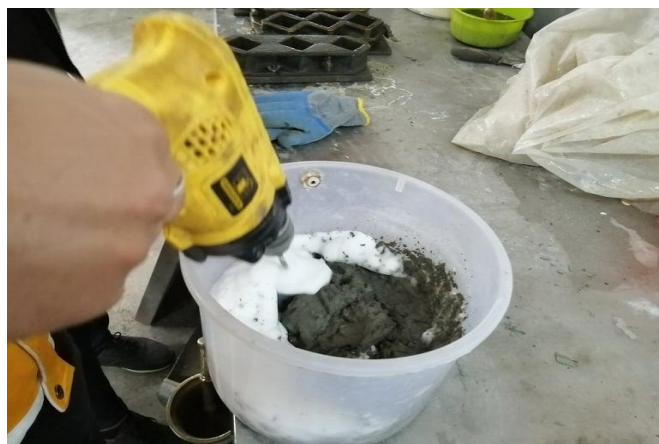
Preparing Foam concrete mixes
